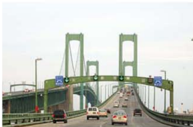
Delaware Memorial Bridge, Wilmington, Delaware
