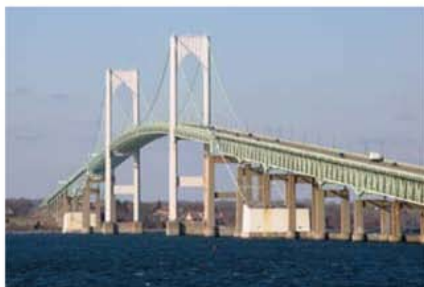
Newport, Rhode Island Bridge
