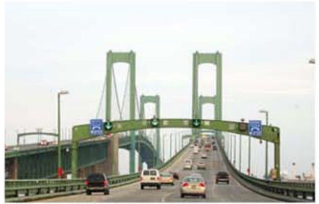
Delaware Memorial Bridge, Wilmington, Delaware
