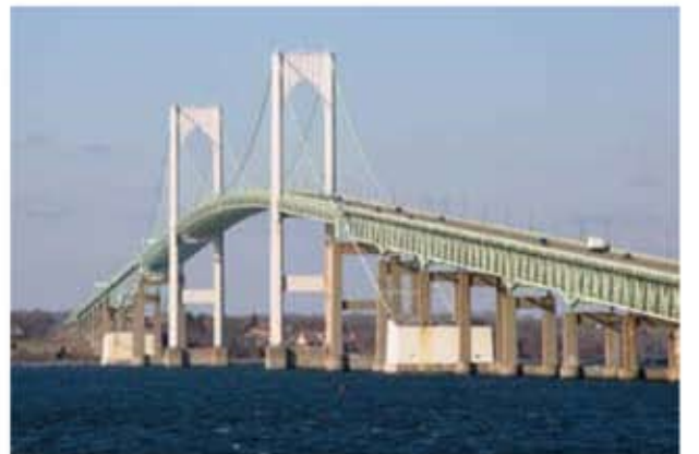
Newport, Rhode Island Bridge
